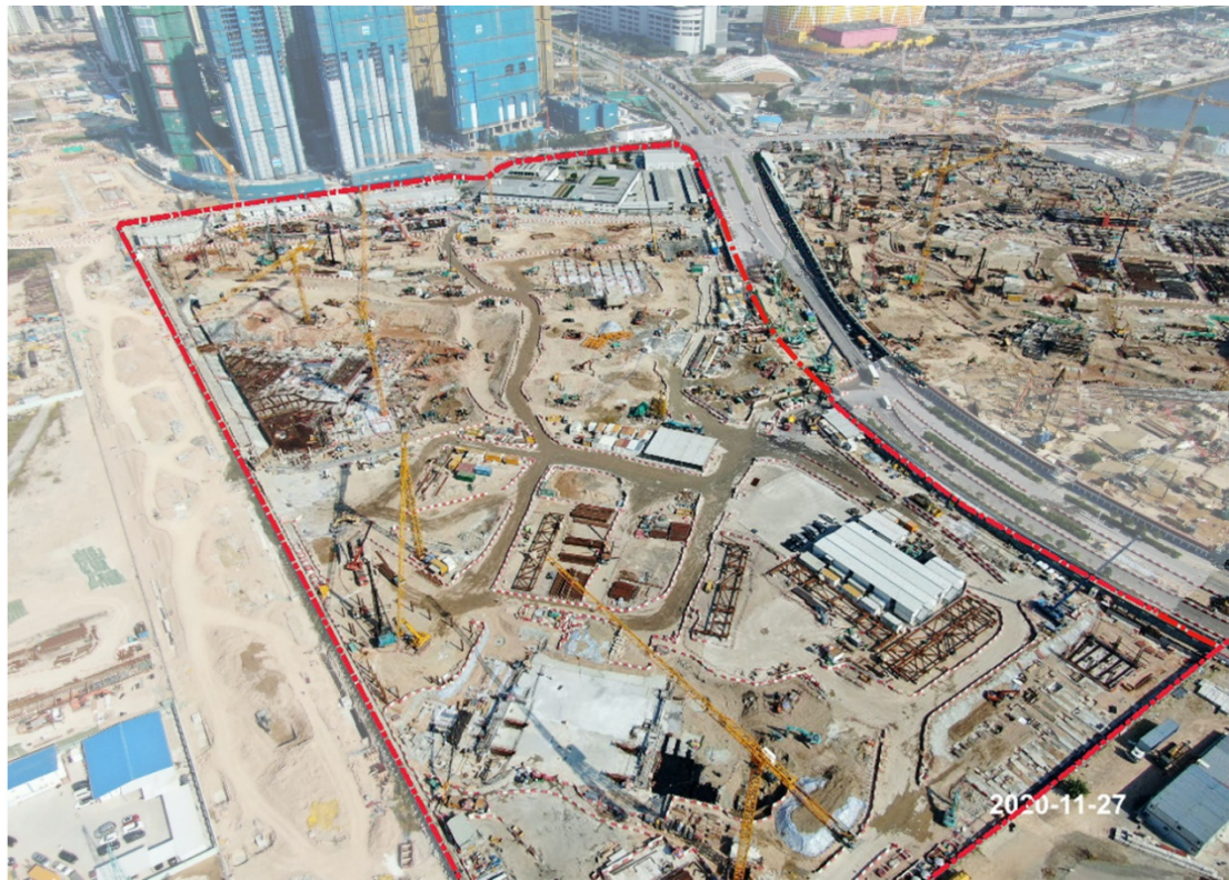
Figure 5: Indoor Sports Centre (top) and Public Sports Ground (bottom) under construction
